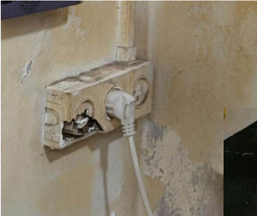
Broken plug socket
